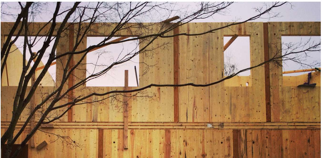
Figure 4.2 Construction of CLTHouse © atelierjones
